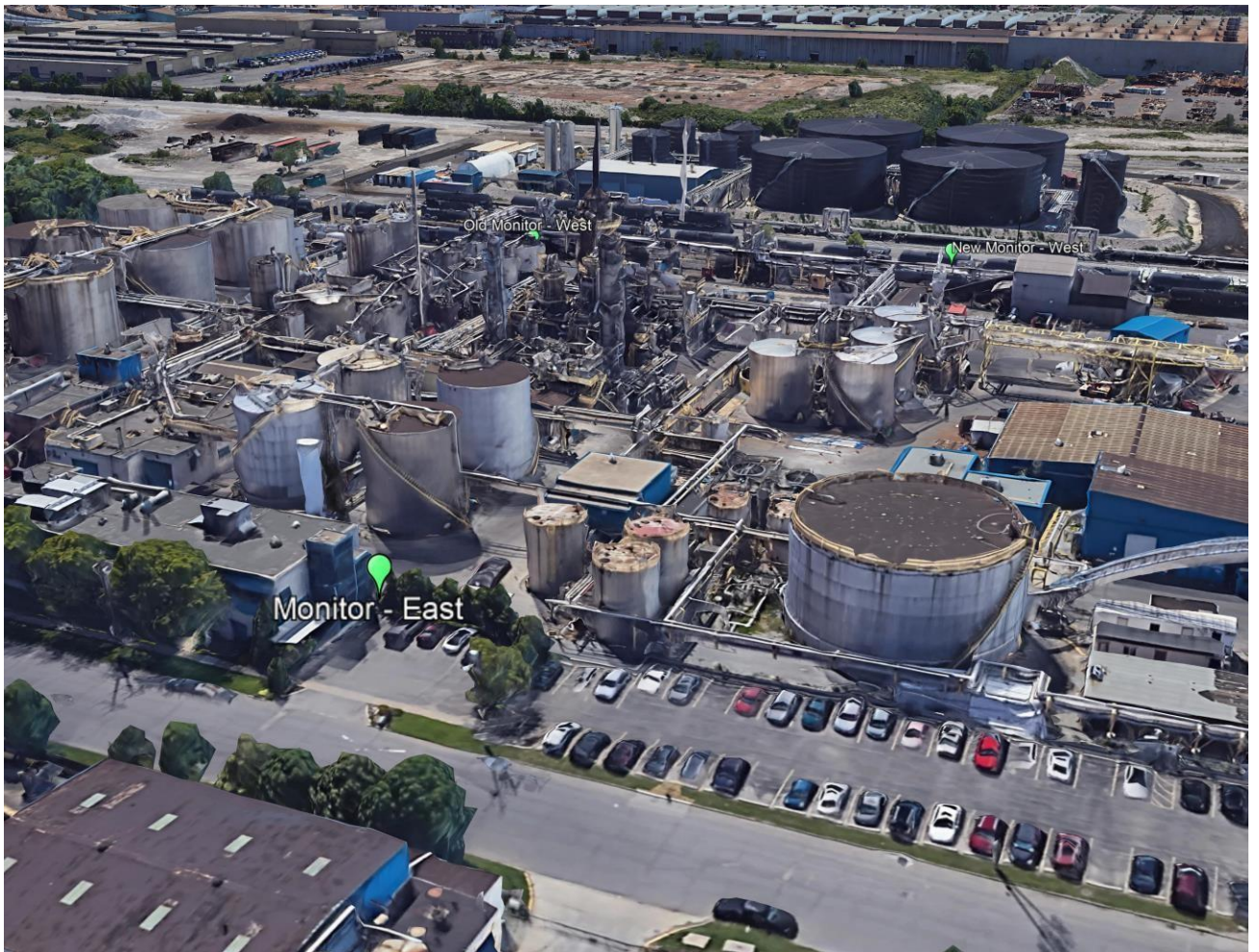
Figure A4: Aerial View 4 – East Monitoring Station
