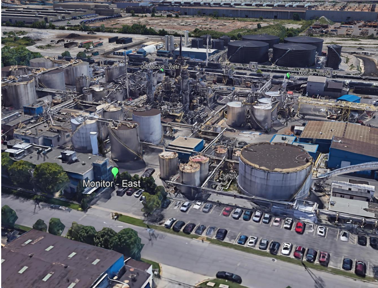
Figure A4: Aerial View 4 – East Monitoring Station
